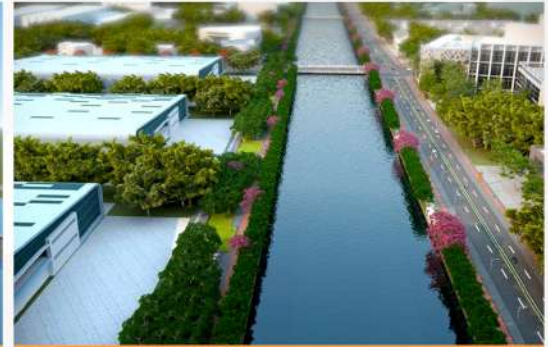
Water Side Area
